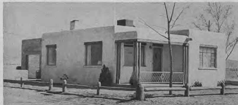
Here is the home of Mr. and Mrs. Harold Cripe which they built with their own hands. They are still working on the home and are about to complete the new garage seen at the left.
