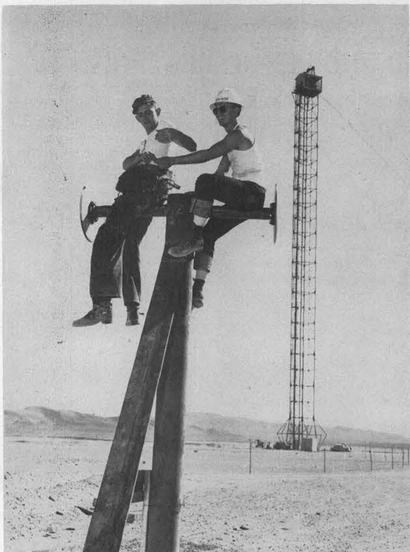
SANDIA LABORATORY'S JOB at Nevada is depicted in part with this illustration of instrumentation men installing gauges which help make pressure measurements of Proving Ground nuclear detonations. In the background is the tower atop which the nuclear device is exploded. Men of the Proving Ground Department pictured here are, Trevor C. Looney, left, and Arnold D. Thornbrough.
