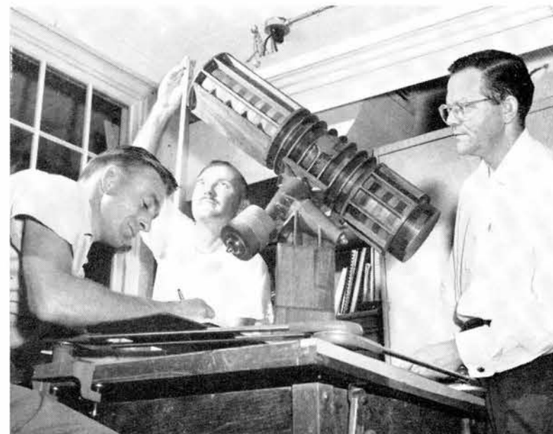
PLANET MARS will be tracked by members of the Sandia Corporation Optical Development Section, 5221-1, in September. Above is a quarter-scale model of the 24-inch tracking telescope which will be calibrated by the sighting the planet when it comes within 35 million miles of the earth Sept. 7. L to R: C. A. Coonce, Dan Parsons and Dan Fenstermacher who are designers of the telescope.
