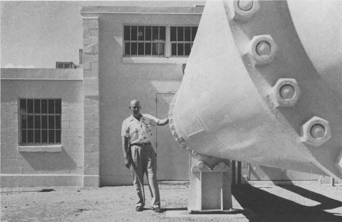
SILENCER to the roar which accompanies tests is this diffuser which extends beyond the building housing the wind tunnel. Cecil Tolbert stands at the far end of the tube which carries the air.
