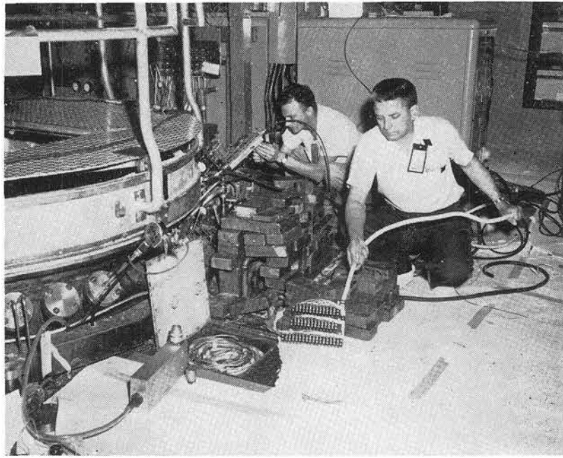
JIM SISLER (5432), right, and a Phillips Petroleum employee work on circuit wiring for a dynamic radiation effects test of electrical devices in the Idaho Falls Materials Test Reactor. The devices, not shown, will be lowered in a special container into the reactor high neutron flux area for irradiation. Instrumentation will record performance while the devices are undergoing the bombardment.
