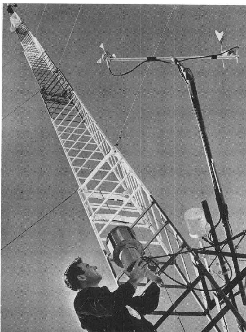
HUMIDITY sensor at 12-ft. level of 100-ft. SMILE tower is checked by Al Brazda (7243-2). Network of seven towers provides weather information for the Albuquerque Area.
