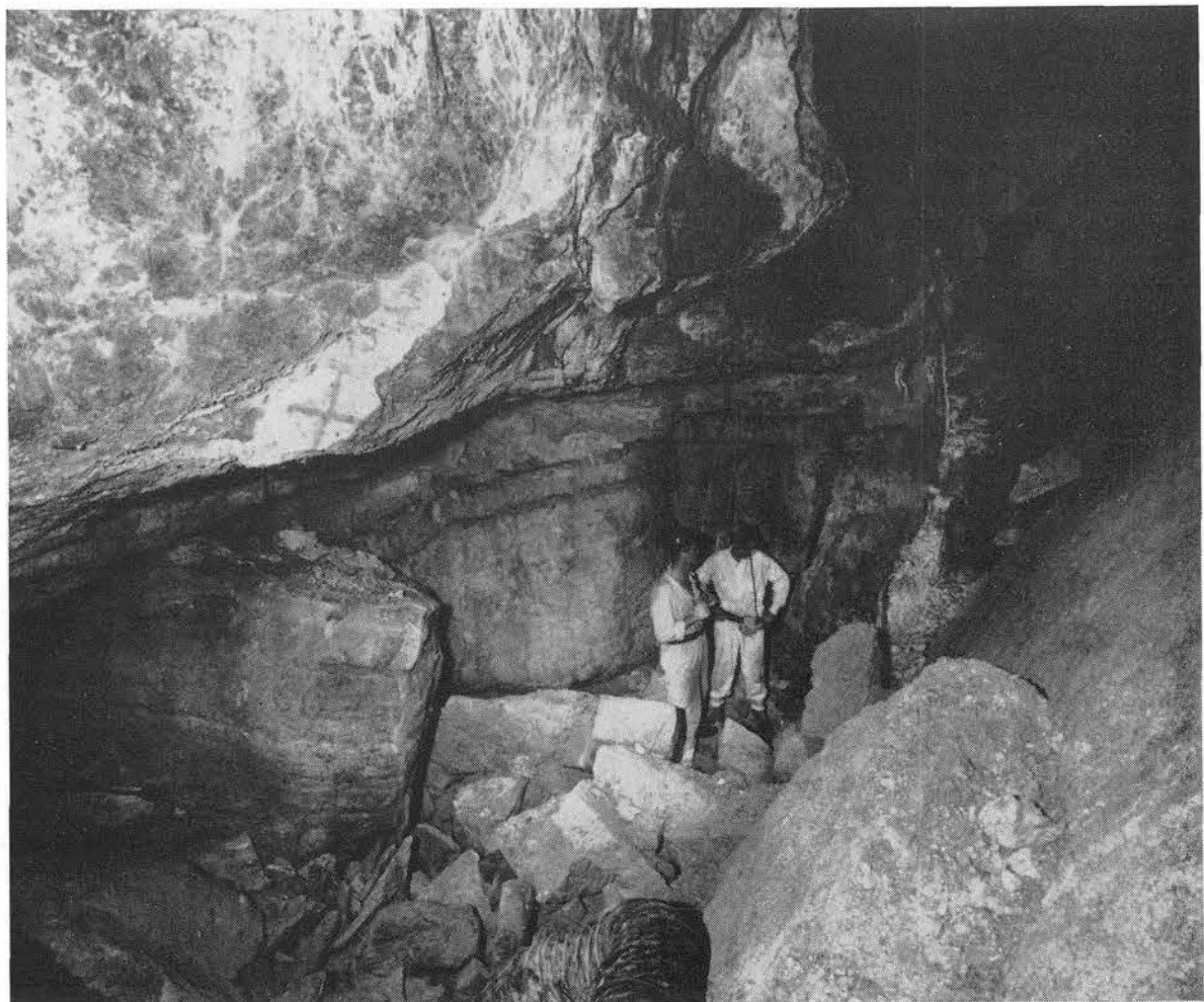
GNOME CAVITY, 1200 ft. underground, now has a general radiation level of 5-15 milliroentgens per hour. Shown here is the entrance of the cavity. The project
