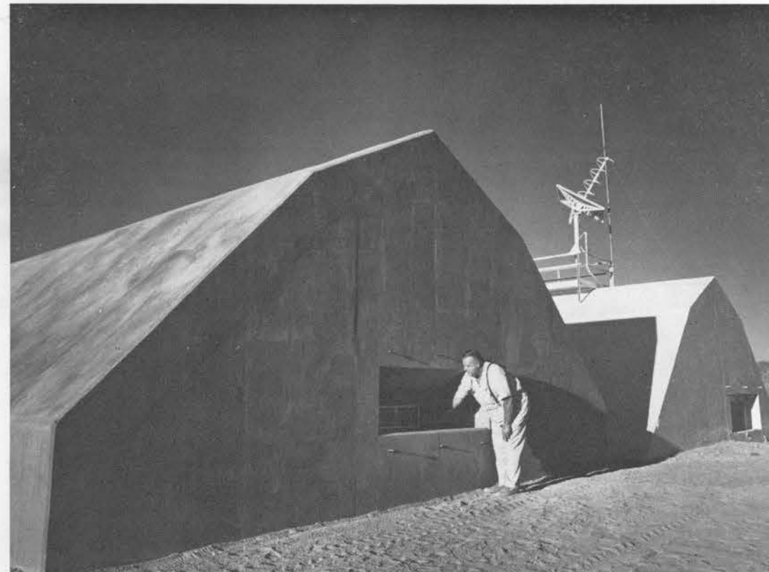
NEW BLOCKHOUSE at Tonopah Test Range is inspected by R. C. Holland, Rocket and Ordnance Section. The new building will house all instrumentation needed to fire rockets from nearby launchers. Older blockhouse in background will be used by observers during firings.
