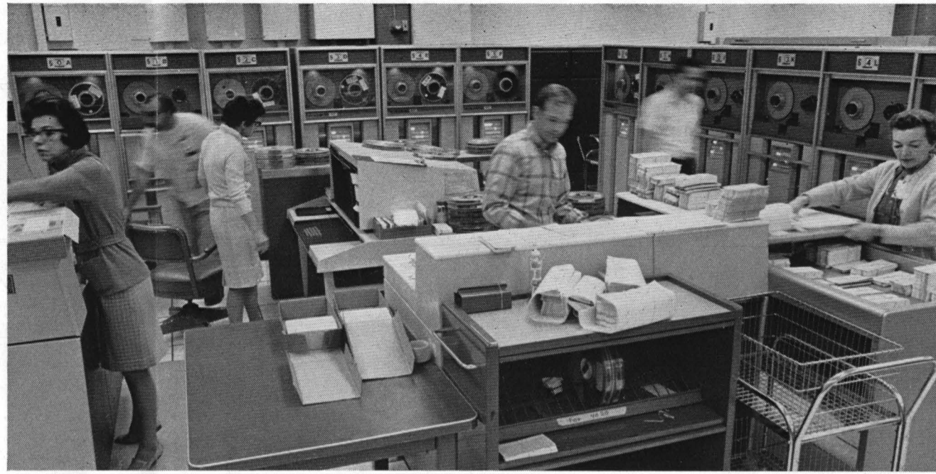
WHERE THE ACTION IS — This busy place is the present 6600 computer console area where operators communicate with the machine, change tapes or perform needed services on the various printers and card readers.
