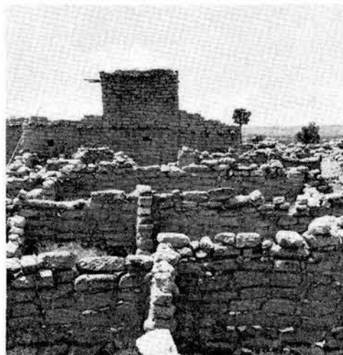
MESA TOP RUINS include multi-storied structures of volcanic tufa block laid in adobe mortar.
