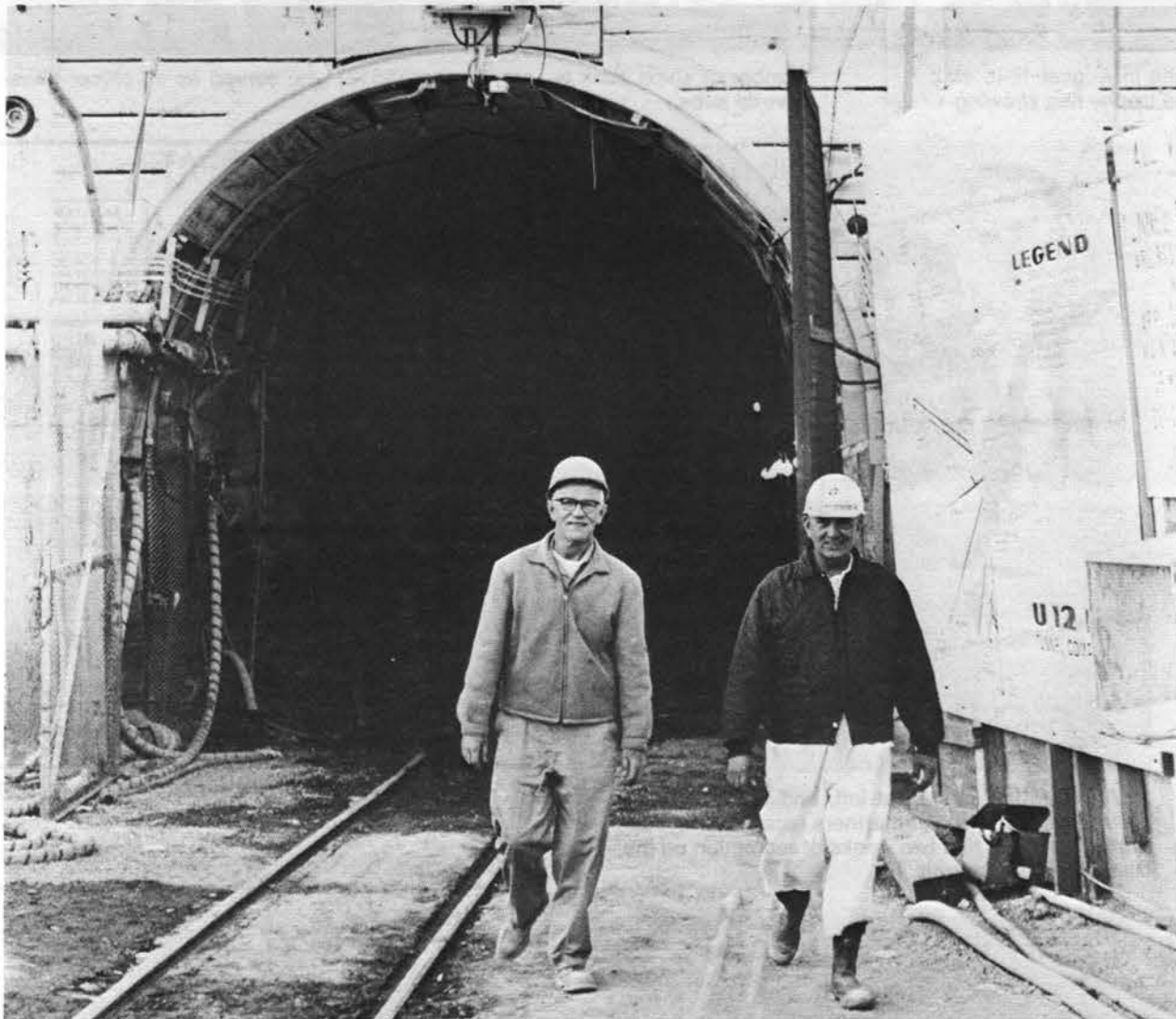
MIGHTY EPIC is the name of an underground nuclear test to be conducted in this tunnel in late spring. Finishing an inspection at the site are Sandia NTS engineering and construction men Al Purington and Smokey Byrne (both 1131).
