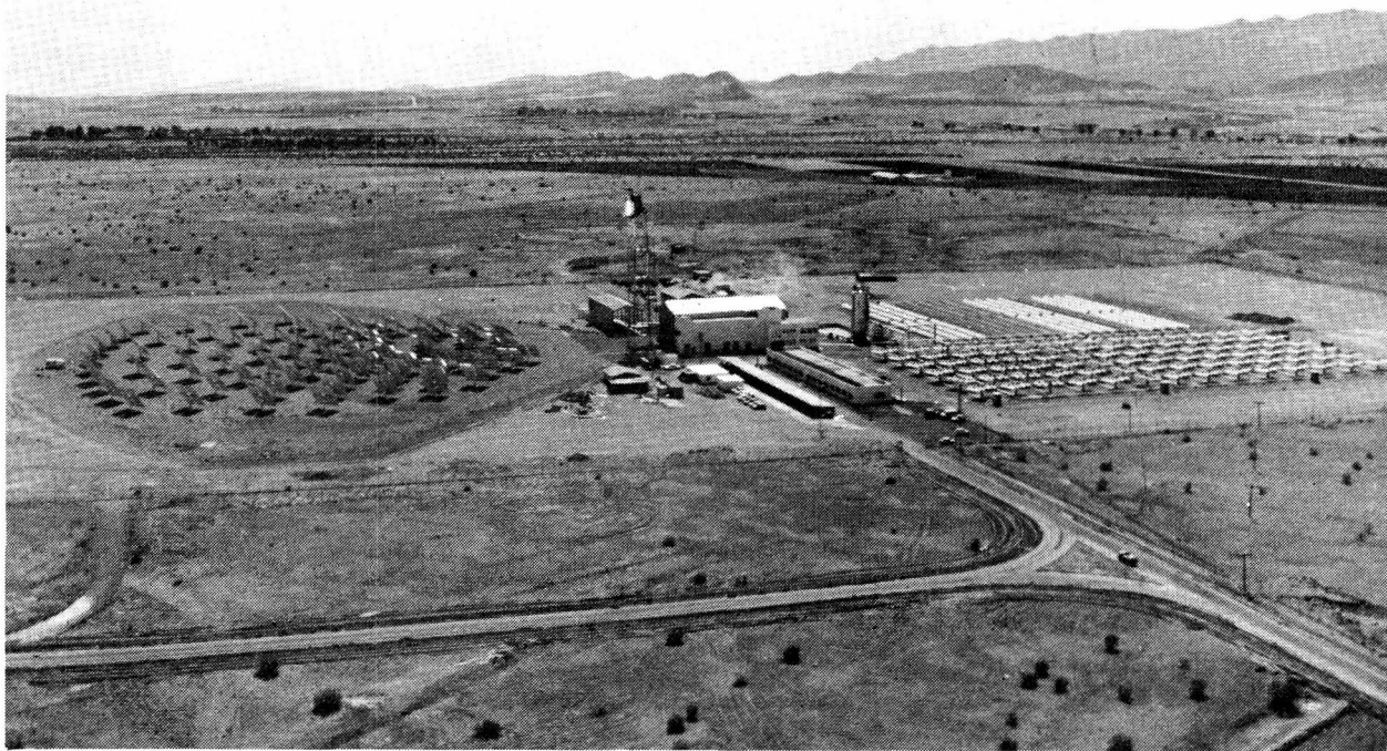
SOLAR ENERGY project at Almeria, Spain, with solar central receiver system at left, distributed collector system field at right.
