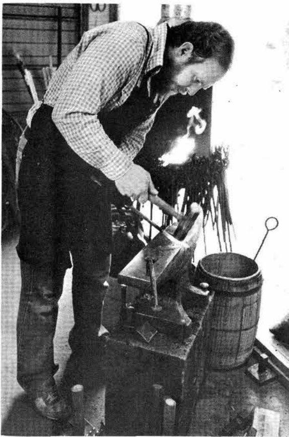
BLACKSMITH AT WORK —Both the forge (in background) and the 100-year-old anvil were located through a LAB NEWS "wanted" ad. Robb Gunter made most of the tools hanging in the rack around the forge from steel auto springs found in a junk yard.
