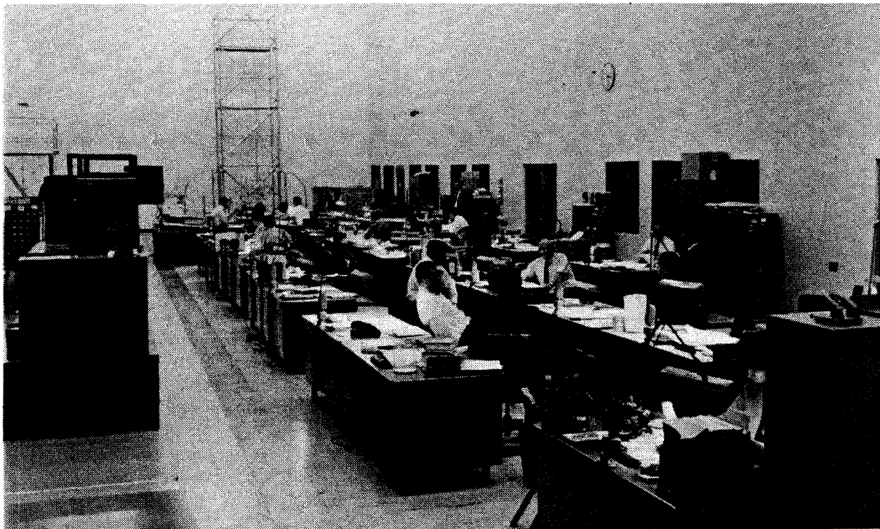
High Bay Area at 50 Danbury Road, Wilton, CT in 1965-66
