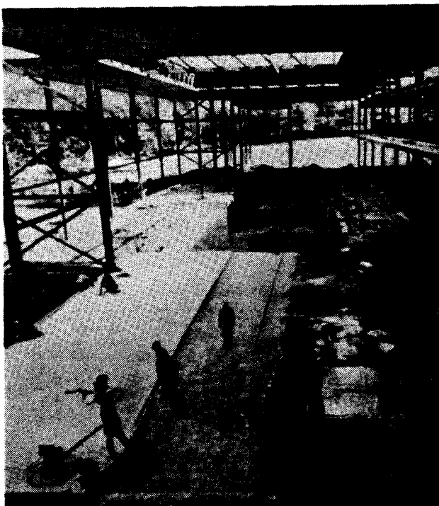
Wooster Heights Facility Construction
