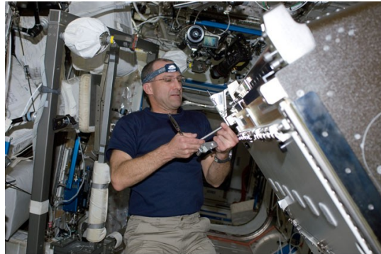
S126E-008178 (18 Nov. 2008) --- Pettit installs the Water Recovery System (WRS) rack in Destiny lab.
