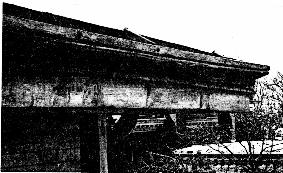
Severely Deteriorated Gutter and Cornice at Dome Eave
