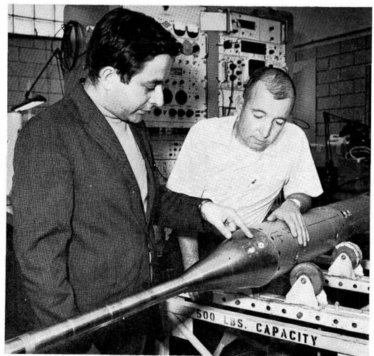
NIKE-APACHE ROCKET will carry this instrument package during the forthcoming high altitude density test series in Hawaii. K. J. Touryan (9326) is showing J. P. Gallagher (9323) location of a new measuring device, an electron beam, which will be used in addition to a pitot-static probe.
