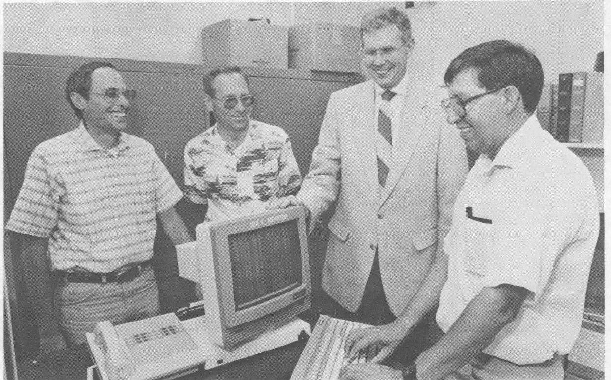
OPERATION OF NEW PBX SYSTEM is reviewed by (from left) project leader Spencer Nelson (2647); Larry Tolendino (also 2647), who assisted in designing the system; Computing Director Larry Bertholf (2600); and Joe Sena (2648-1), who will complete its installation. The new system has already been installed in Area IV and in parts of Bldg. 880. Installation throughout Sandia should be complete within a year.
