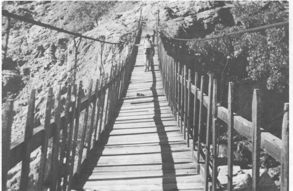
CAUTIOUSLY CROSSING a Hollywood-style foot bridge on the road to Satevo, Mexico, is Trudi Martinez, Gene Roseth's (9242) traveling companion. Gene replaced missing planks and tested rotten wood before crossing over to take Trudi's photo.
