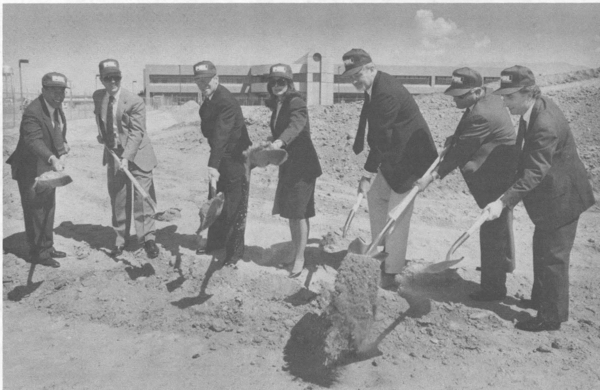
BREAKING NEW GROUND: Sandia research in materials sciences will be housed in the Integrated Materials Research Lab, south of the Microelectronics Development Lab (Bldg. 858, background). Wielding the shovels are (from left) Ricardo Zuniga, Project Specialist for US Sen. Jeff Bingaman; Bruce Twining, Manager, DOE Albuquerque Operations Office; US Rep. Steve Schiff; Linda Alvarado, President, Alvarado Construction (contractor for the IMRL); President Al Narath; Vice President-1000 Venky Narayanamurti; and Paul Gilman, Administrative Assistant to US Sen. Pete Domenici.
