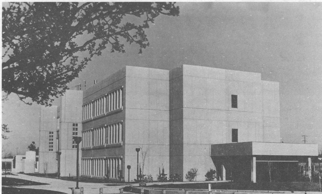
COMPLETED THREE years ago, Bldg. 910, the Weapons Laboratory, has three floors and a basement, which together total 85,000 square feet.
