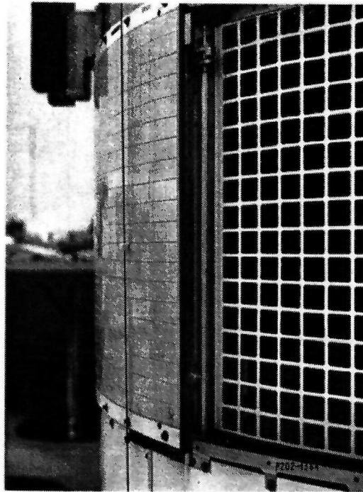
Fig. 7. Slot-feed transformer.
