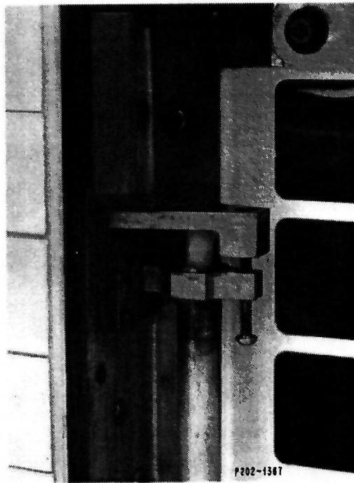
Fig. 9. Adjustable shunt capacitor.
