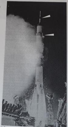
A Soyuz A-2 launch with two vital elements of the T-10 abort indicated. The upper arrow shows the rockets of the escape system; the lower points to the 'petals' that were deployed to slow down the escaped craft. (This picture is from the French/Soviet mission of June 1982).
